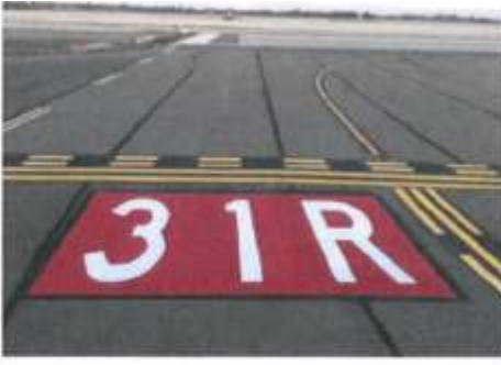
Surface Painted Holding Position Marking
